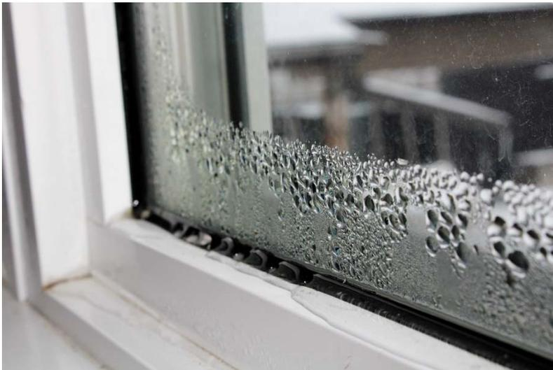
**Windows** – Bad window seals can lead to moisture intrusion into the building. Additionally, condensation on windows can result in mold growth.
